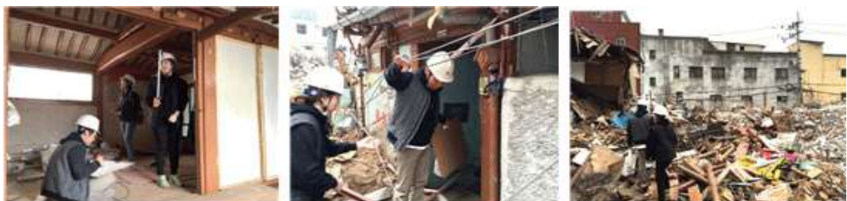
Figure 14. Photos of traditional housing for Store(Muakdong 46-15)
